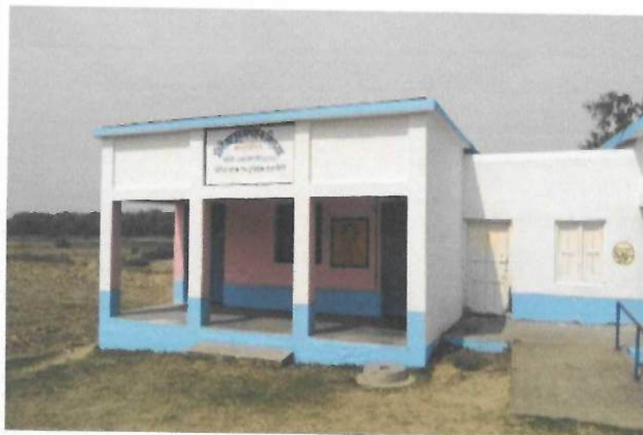
Completed painting work for Nidhirampur Primary School
