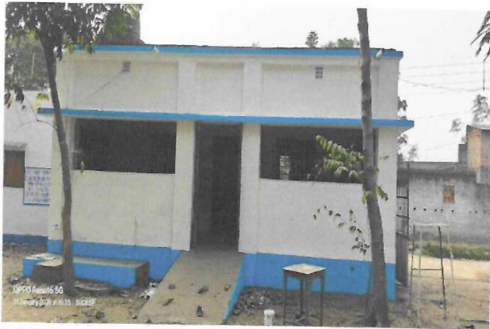
Dumuria Primary School painting work in progress
